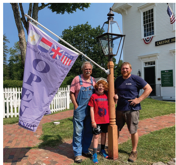
Marc Pelletier, Hollis Skillen, and Steve Skillen installed a new lamp post in front of the Abbott School. As seen in two photos on this page, young volunteers are crucial!
