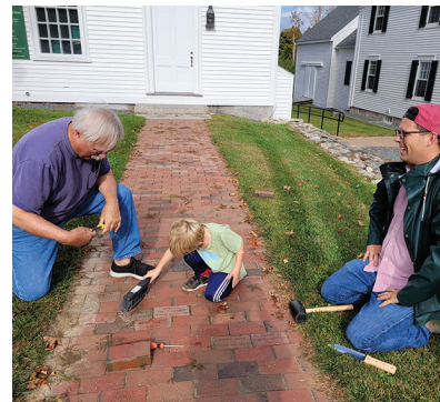
Marc Pelletier, Teddy Pearce, and Charlie Pearce installing engraved bricks
